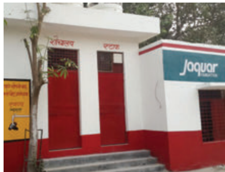
New toilet block for a Government School, constructed by Jaquar Foundation
