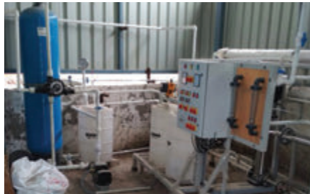
RO Water Plant installed by Jaquar Foundation at Alipur village
